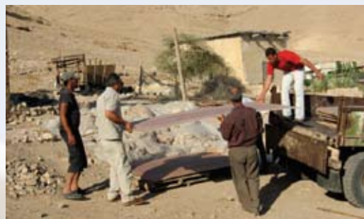
Save the Children UK and its local partner renovated houses for 30 families in the Jordan Valley as a means to prevent forced displacement. PHOTO/Hiba Qaraman
